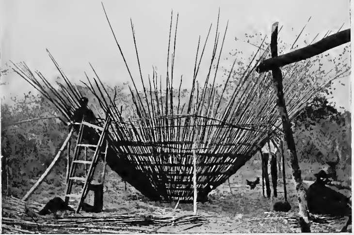
BUILDING THE ROOF OF A HUT.
